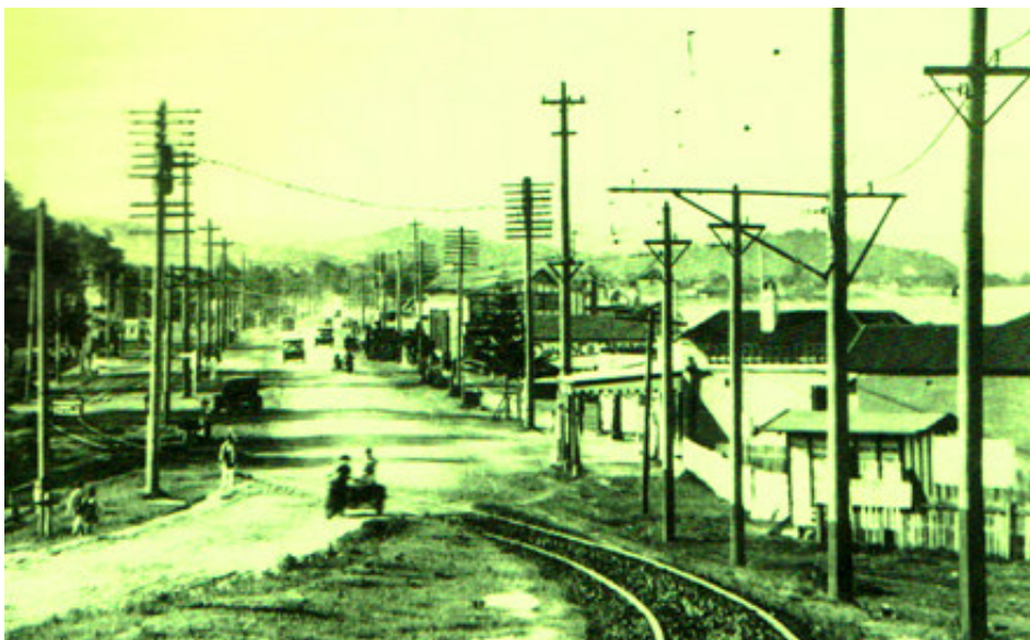
Collaroy shops and tram line.
